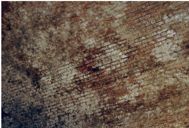
Early Wood Burning Locomotive Exhaust Partially Covering White Washed Tunnel Roof.
