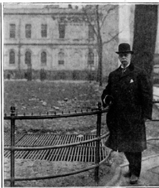
The grating in City Hall Park, covering a ventilating opening leading to the Scientific American tunnel.
